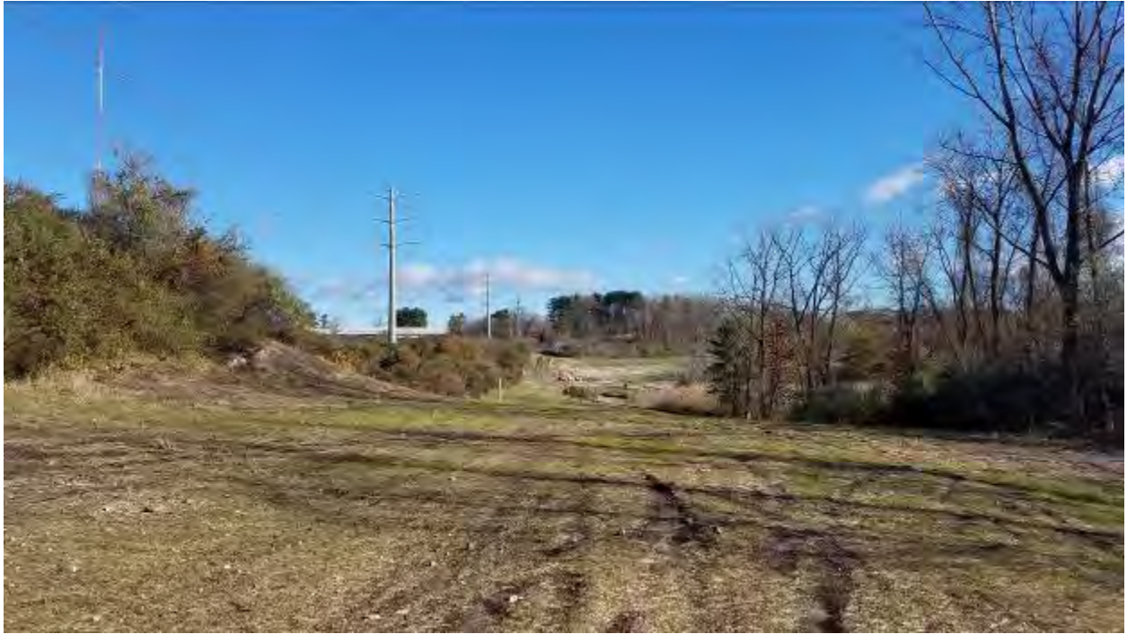
Gas Pipeline Route and Adjoining Property (Looking North)
