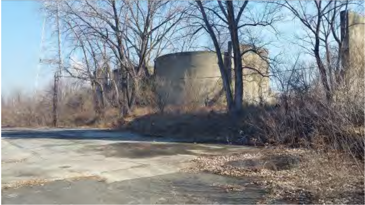
Existing Concrete Silo (Adjacent to Con Edison Retained Parcel 1)
