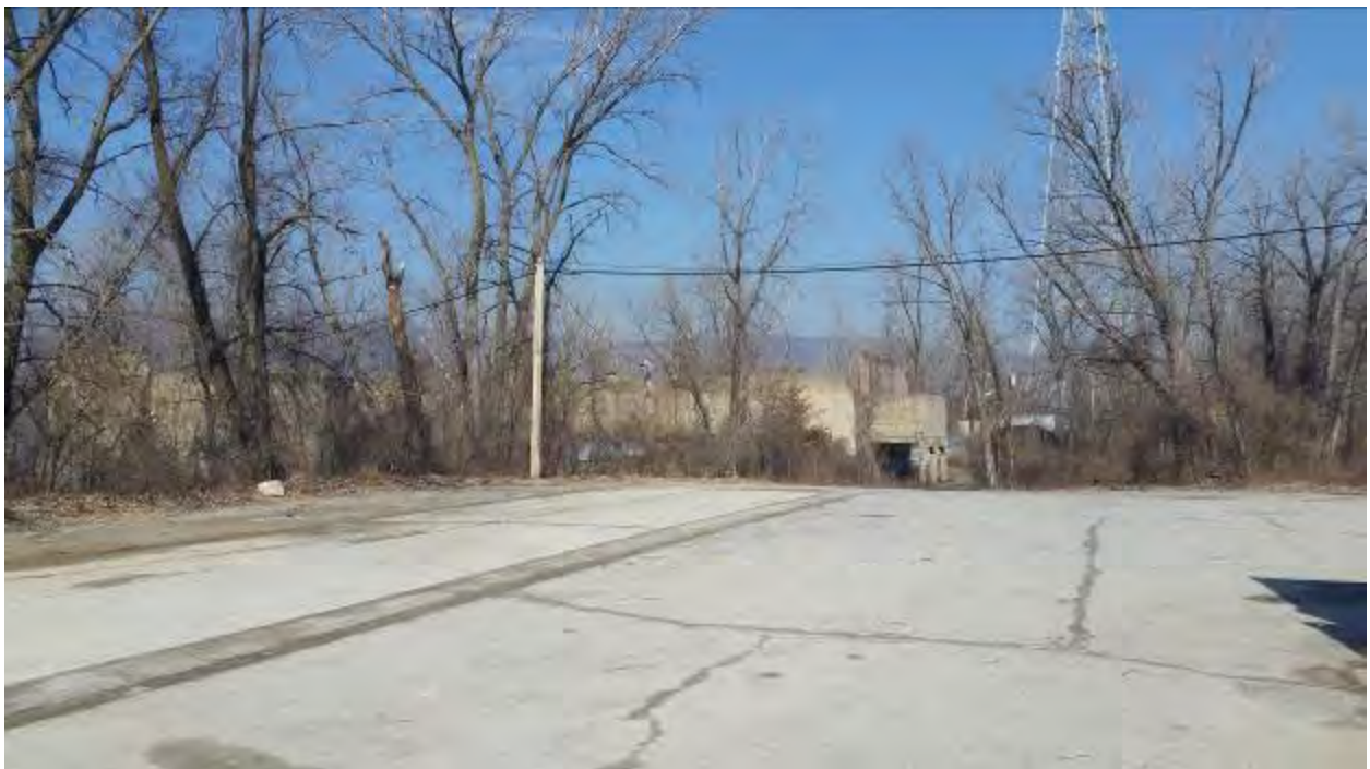
Existing Asphalt Pavement (Area of Merchant's Daughter)
