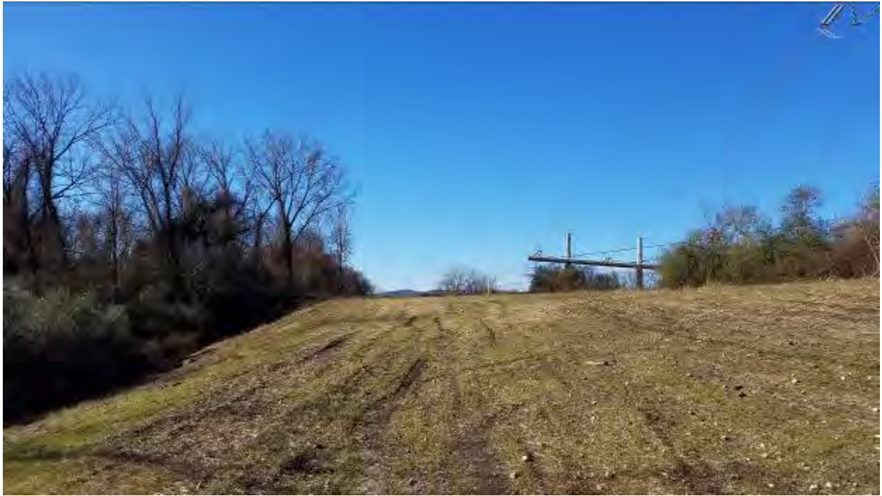
Gas Pipeline Route and Adjoining Property (Looking South)
