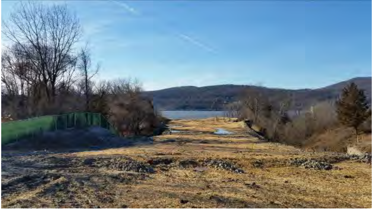
Gas Pipeline Looking West from 11 th Street (Potential Access Road to Riverside)
