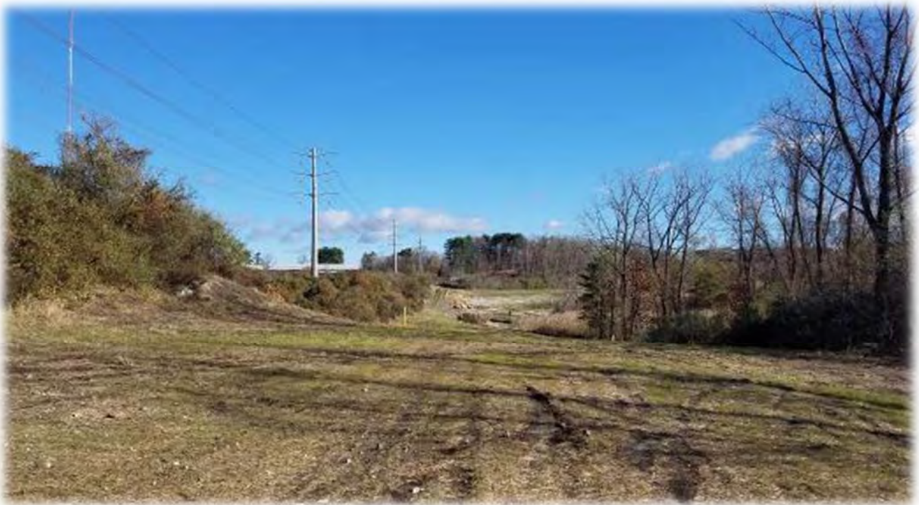
Portion of Site Disturbed for Gas Pipeline
