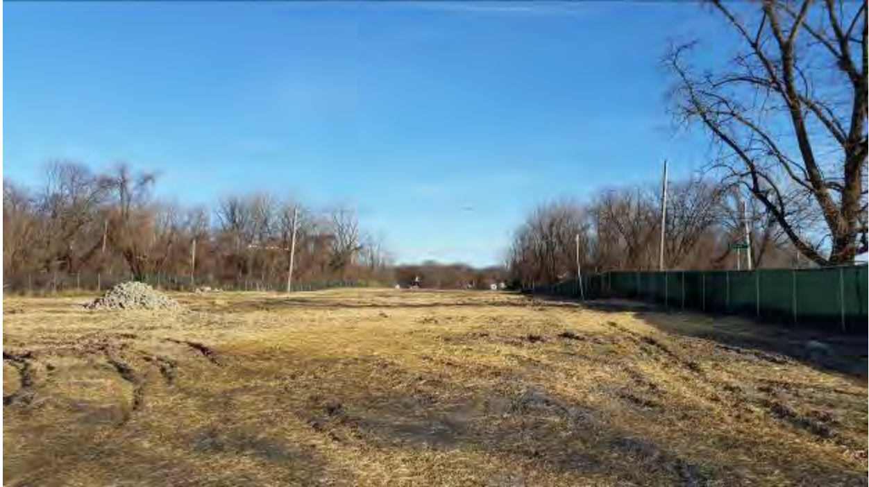
Pullback Area for Gas Pipeline (Highland Avenue)
