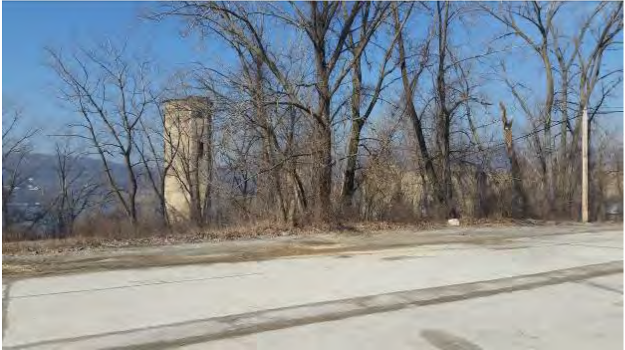
Existing Roadway From Lower 9 th Street (Area of Merchant's Daughter)
