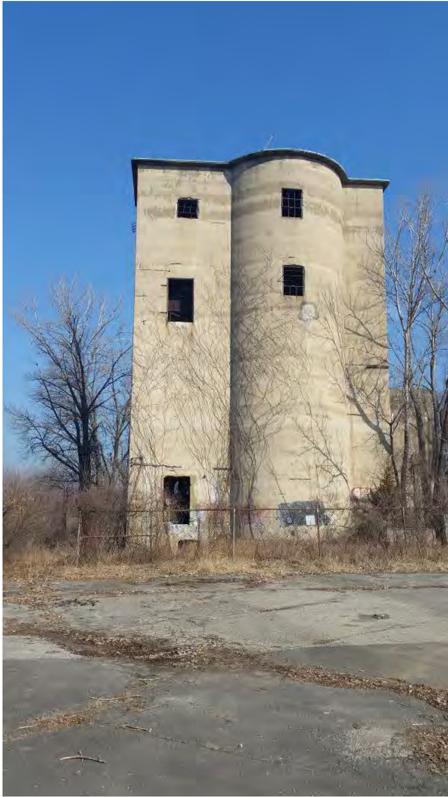
Concrete Silo and Storage Building (Riverside of Quarry)
