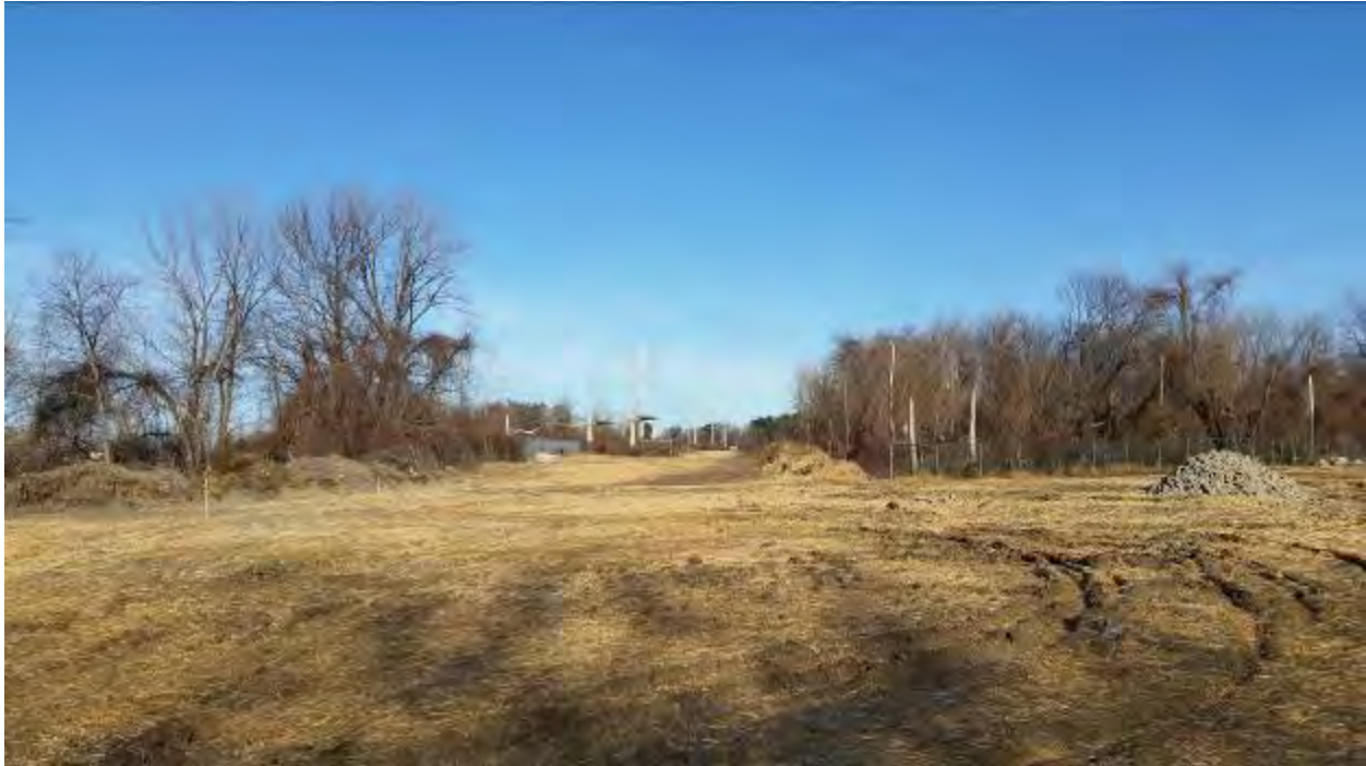
Gas Pipeline Route Looking North from Highland Avenue.
