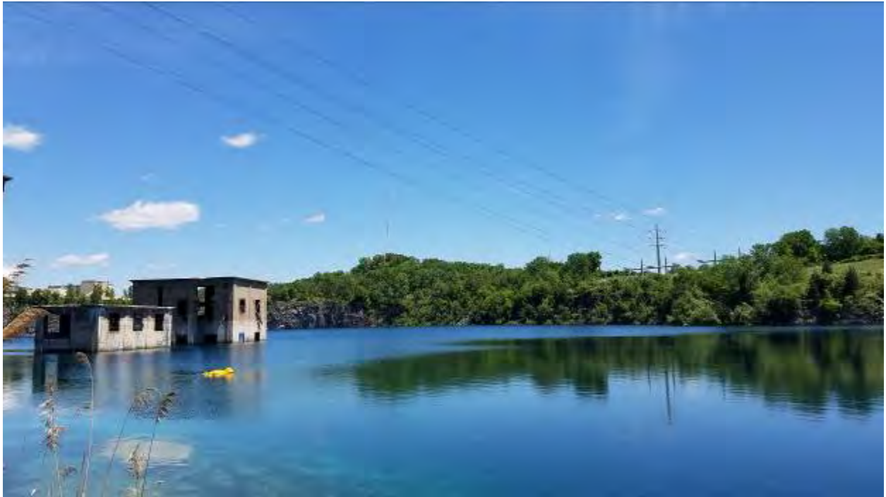
Quarry and Buildings (2019)
